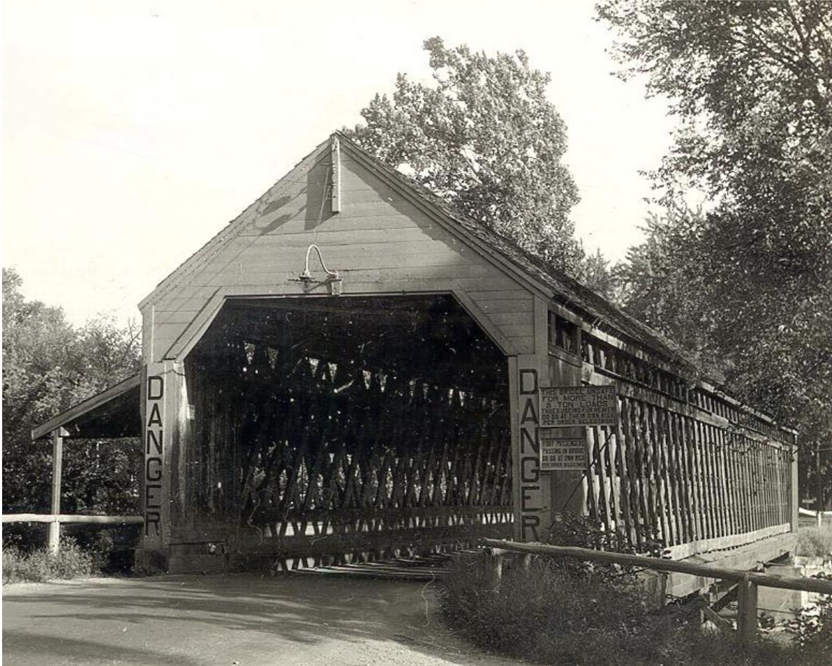
**1962 - 1963** – A new covered bridge is built and dedicated on November 4 1963, named the Chester H. Waterous Bridge after the legislator who won funding for it. The 20 ton capacity pratt truss structure is 184 feet long with 105 feet being covered including two 8 foot walkways.
